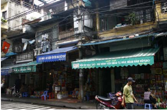
Figure 7: Image of Hang Buom St. before installing unified pent-roof system.
