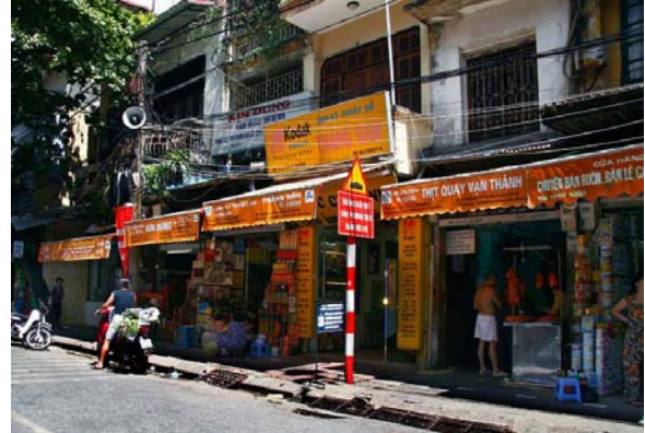
Figure 8: Image of Hang Buom St. after installing unified pent-roof system.
