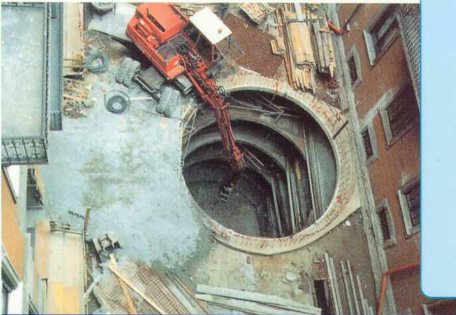
Excavation and execution of the slabs (top-down)
