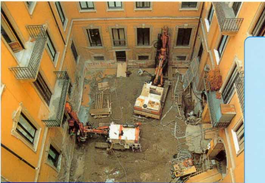
Execution of the retaining structure
