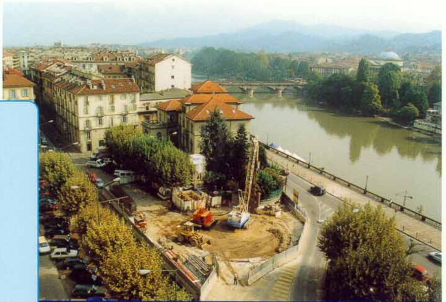
Site area is reduced to the minimum during construction
