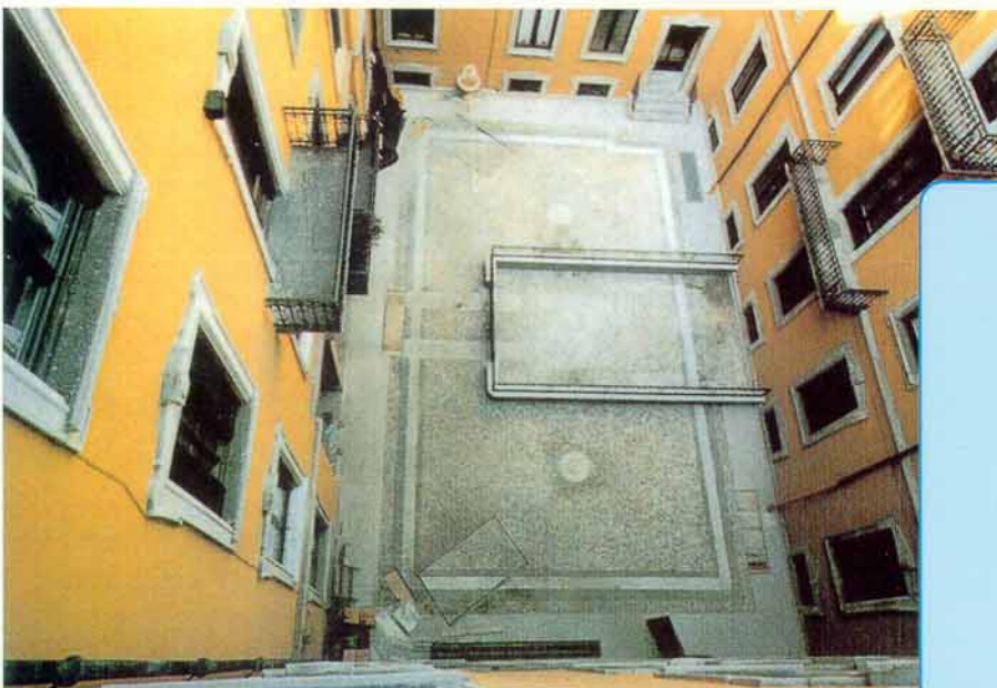
Completion of TREVIPARK structure
