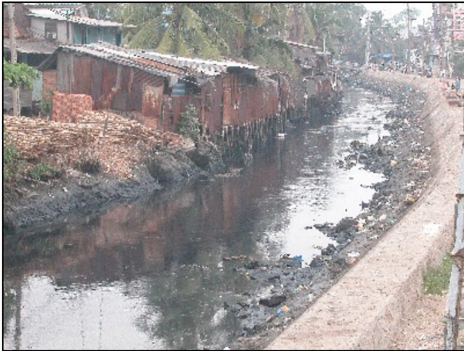
Figure 8: One branch of To Lich River 4
